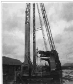
a) Core drilling machine
